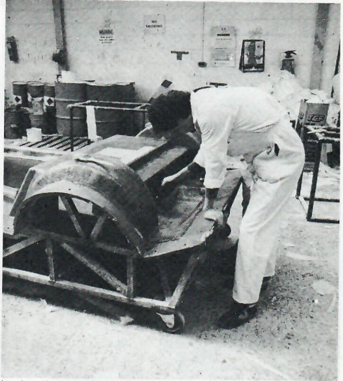
Laying the glassfibre
