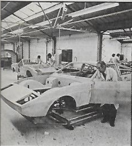
After leaving the moulds the shells are rubbed down and carefully examined for pin-holes. A Coupe is in the foreground and a Convertible behind.
